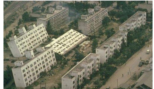
Figure 2. liquefaction damage caused by the 1964 Niigata Earthquake
