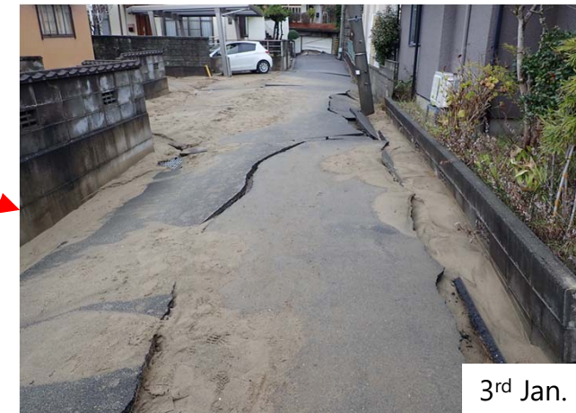
Lower part of the slope: Ejected sand and uplift of sidewalk
