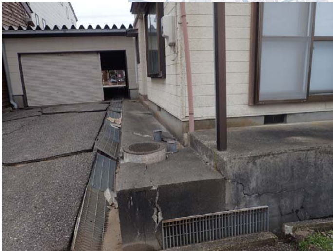
Severe liquefaction damage on residential house
